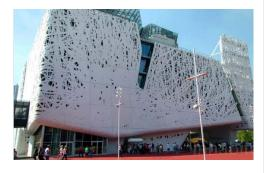
Imagine a building that could eat smog and digest it to harmless substances! Palazzo Italia is the first building designed to clean the air! The construction material used is able to capture pollutants in the air and convert it to non-polluting compounds, which will be rinsed off when it rains!
